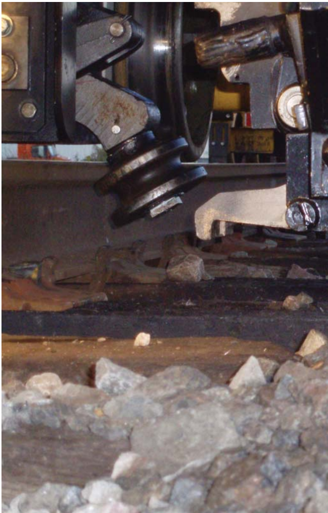
Rail jacks raise the rail while the finger assembly inserts and positions the plate.
